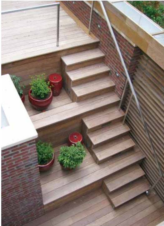
Garage Roof Deck
